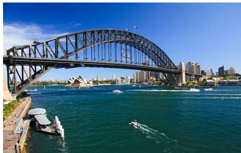
Sydney Harbour Bridge
