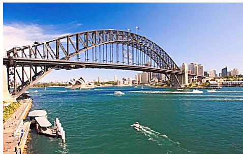
Sydney Harbour Bridge
